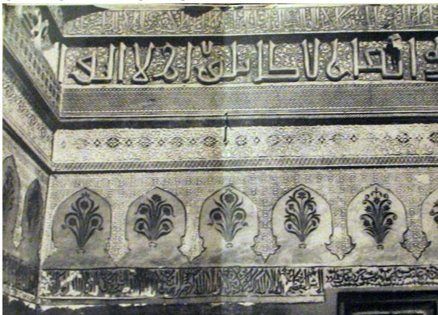
Interior view of Khoja Amin mausoleum
